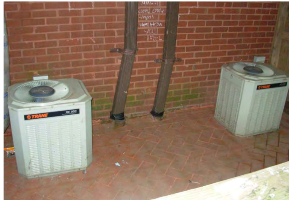
20. Typical HVAC system exterior condensers, some on roof of Chestnut
