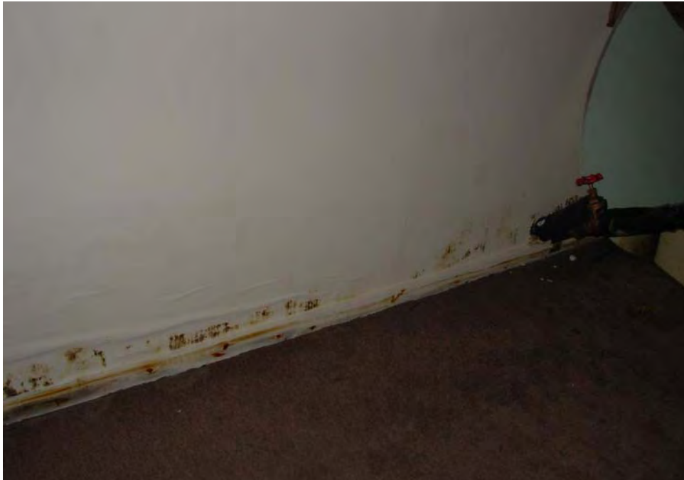
9. Water damage and mold growth at basement of Edwards
