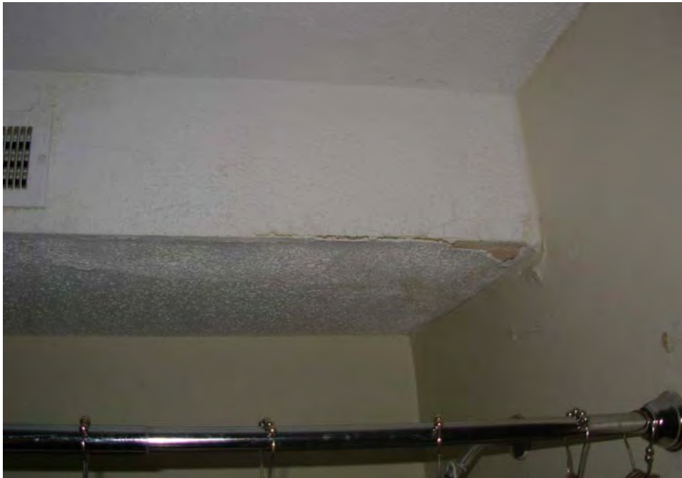
15. Spot wall damage and joint failure observed in units
