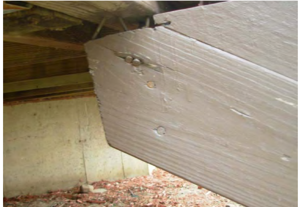
10. Stair framing fatigue at front of Edwards
