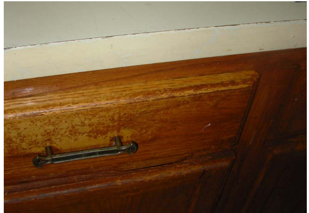
18. Finish wear and some damage prevalent on cabinetry
