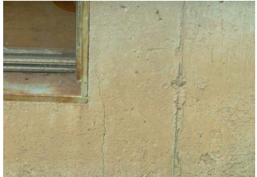
8. Spot foundation cracking observed
