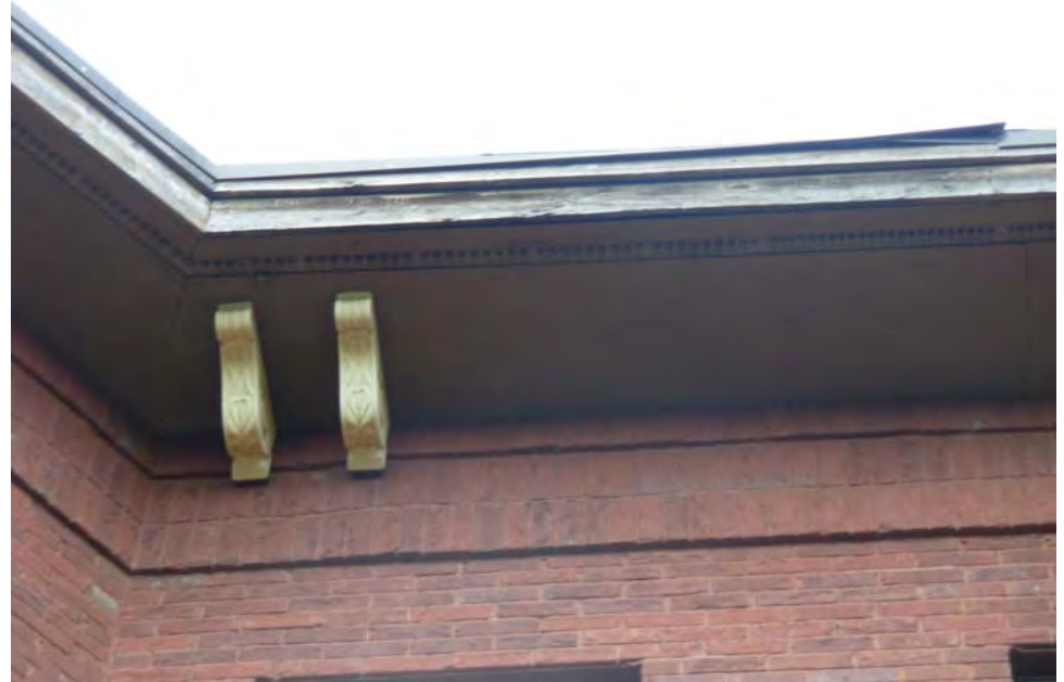
14. Cornice and soffit at both buildings to repair and refinish
